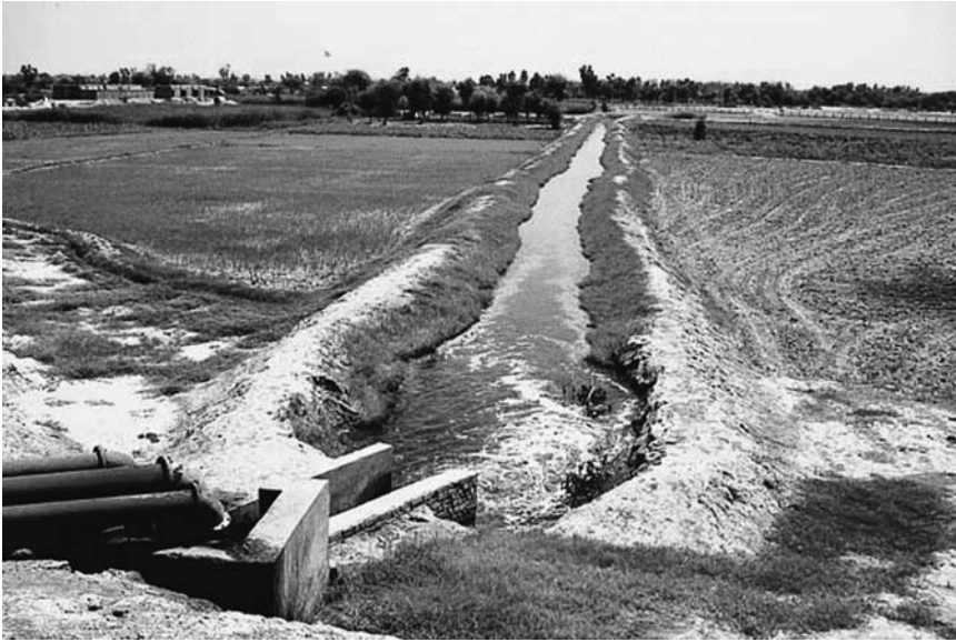
Plate 10.2. Pipes taking untreated wastewater from a wastewater drain before it enters the WSP (Photo: J. Ensink)
